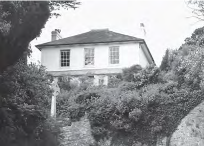
Figure 56 The 'polite' style of this 19th century house derives from the formality of its architectural treatment which creates a dignified and refined appearance
