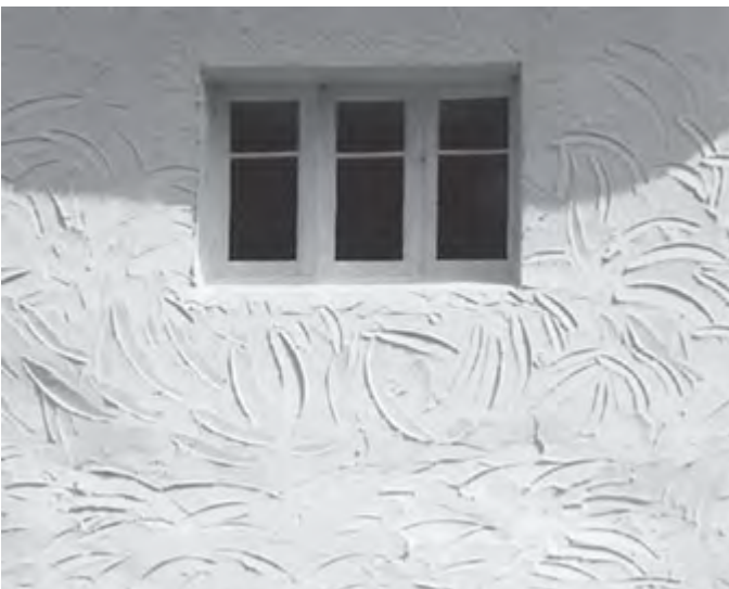
Figure 53 Renewing the render of this cottage was appropriate, but not the added patterning
